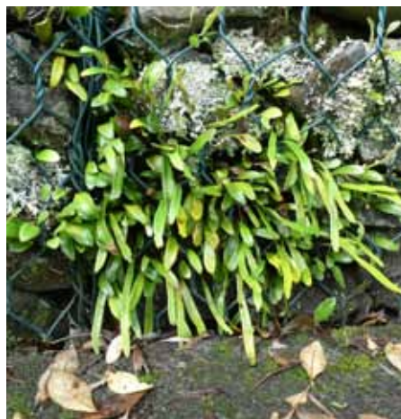
Photo (above): On gabion wall
