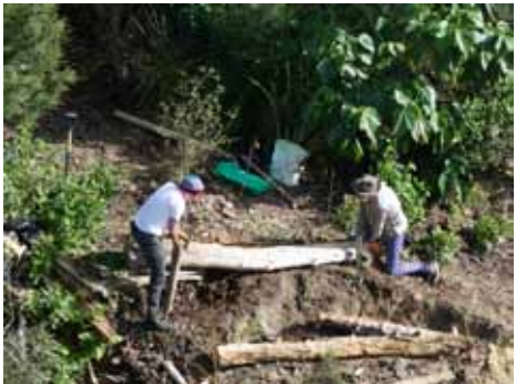
Photo (above): Glenn & Chris building terraces
