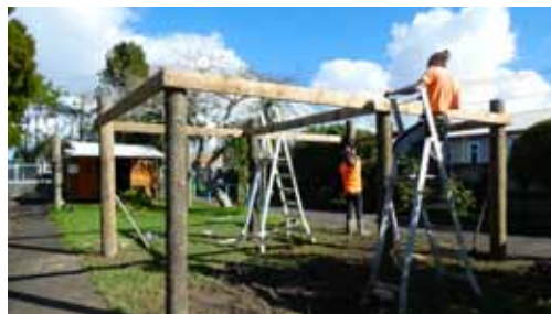
Photo (above): Shade house construction
