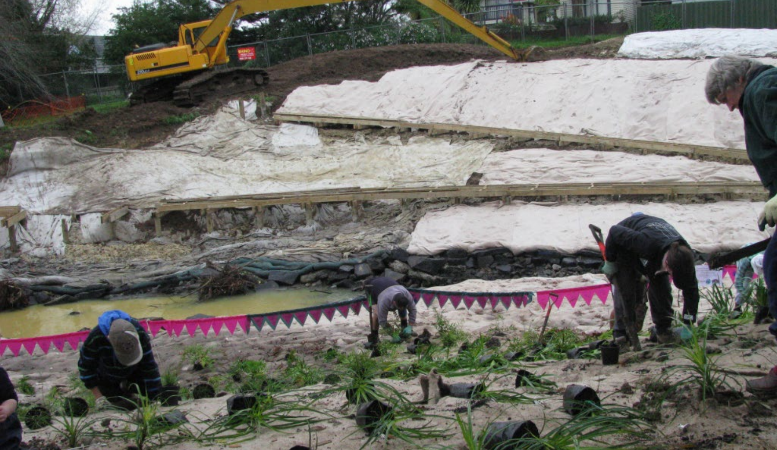
Volunteer planting at La Rosa Stream – managing health and safety
