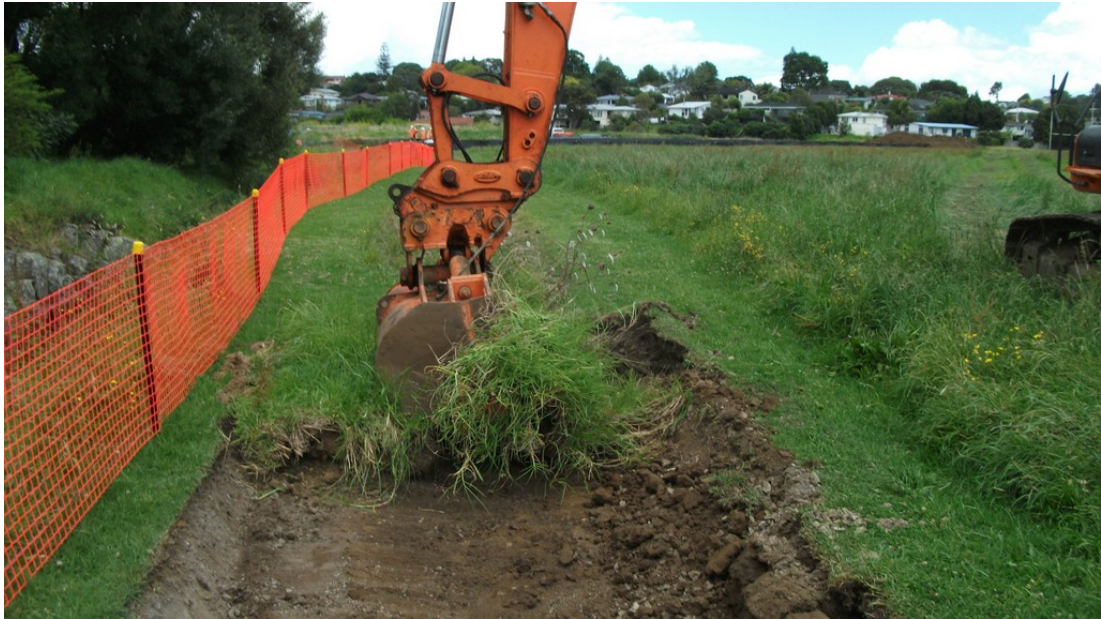
Sod translocation of Geranium "Te Auaunga" along the banks of Oakley Creek.
