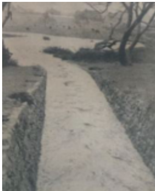
Figure 2. ‘Storm water flowing successfully in the recently widened and deepening section of Oakley Creek, Mount Roskill. This area has always been subject to floods in the past.’ [Picture of flooded stream with cows grazing in background believed to be in the May Road Memorial Park.] Source: New Zealand Herald , 19 May 1954. MRB 127 Newspaper Clipping Book 1954-1960. Part 2. Auckland City Archives.
