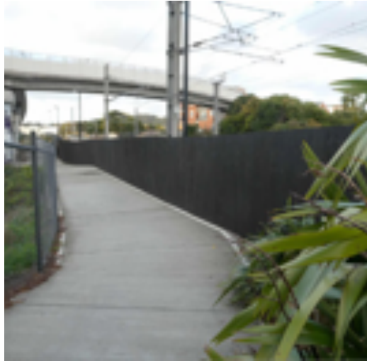
Photo (above): A blank canvas - the black fence running along below Te Arawhiti o Te Wai o Rakataura (Soljak) Bridge.
