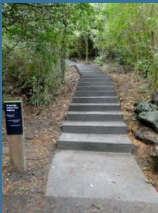
Photo (above): Path Renewals, new steps
