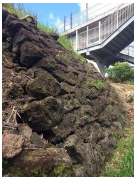
Photo (above): Stone Wall Embankment (Chris Brown)
