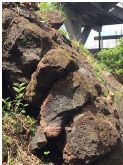
Photo (above): The internal structure of the Embankment (Chris Brown)
