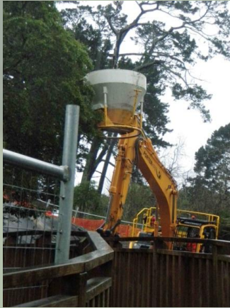
This is how concrete comes in for construction of the bridge foundations. Photos: W. John
