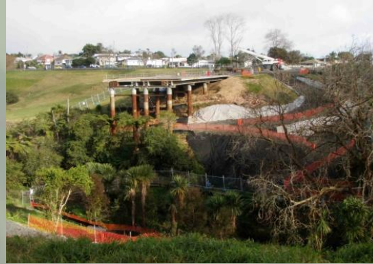
This is how concrete comes in for construction of the bridge foundations. Photos: W. John
