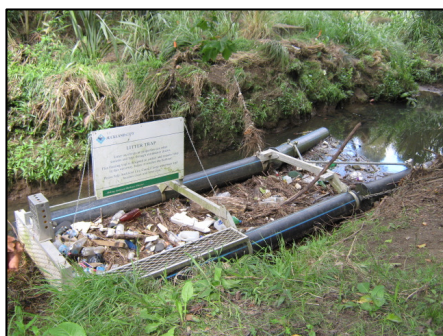
Figure 7: Floating Litter Trap (NT1416) in Oak_3, Oakley Creek
