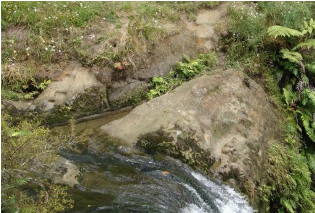
Plate 16. Western bank of waterfall with cut channel in bedrock visible with fern growing within it.
