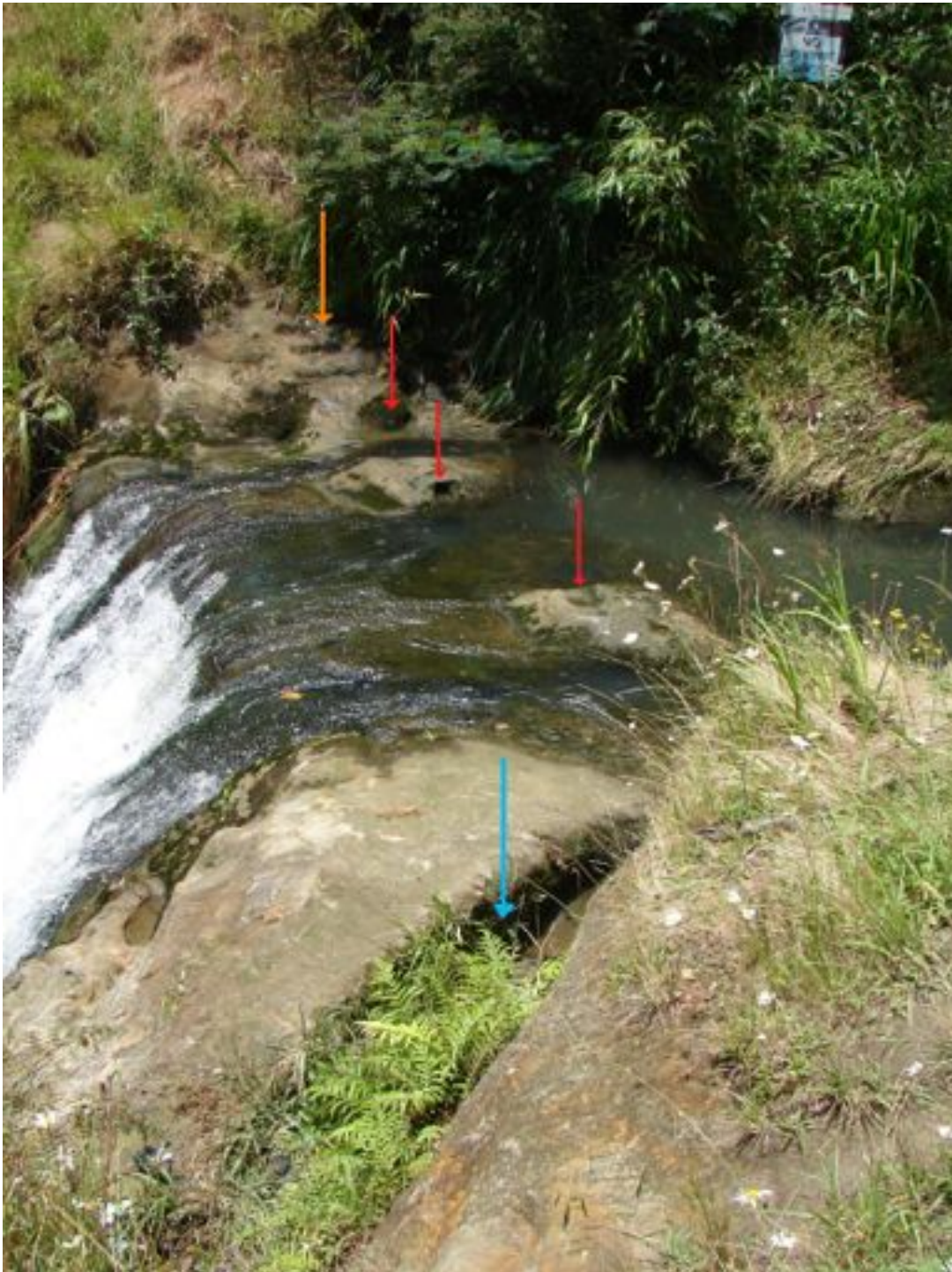
Plate 17. Top of waterfall with cut channel in bedrock visible with fern growing within it (blue arrow), cuts for posts across top of falls (red arrows) and steps cut into bedrock (orange arrow).
