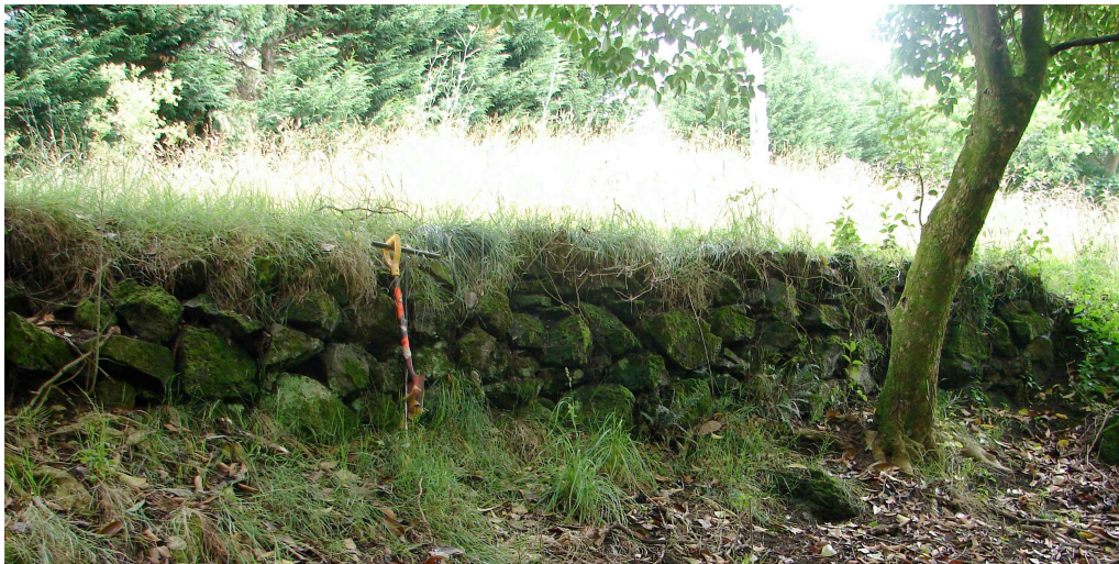
Plate 9. R11/2473 illustrating close proximity of a tree.
