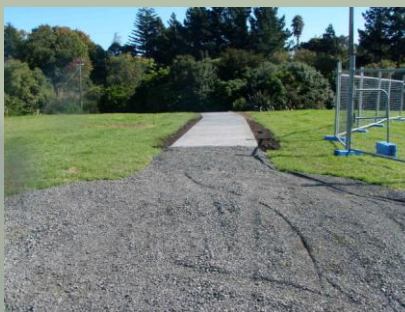
Above: The Harbutt path connection has been completed. The gravel at the front (left) is a temporary surface until the Waterview Shared Path is built and the two are connected. Photos: W. John
