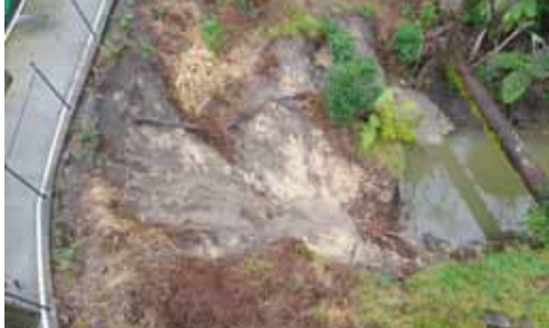
Photo (above): Slip at Railway Heritage area also revealing soakaway pipe (Gina Hefferan)
