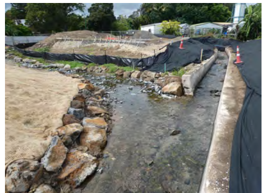
Photo (above): Work to daylight the Wairaka Stream
