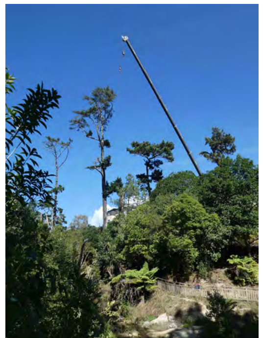
Photo (above): A very tall crane was needed to clear the fallen pine away
