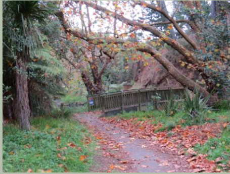
Plane Tree Bridge
