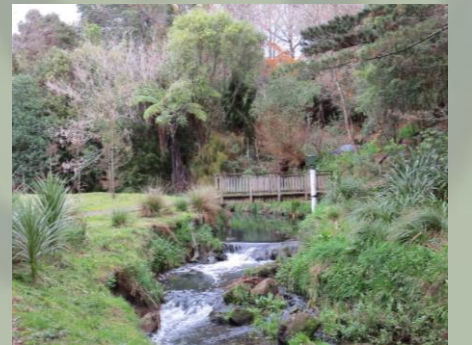
Cradock St Bridge
