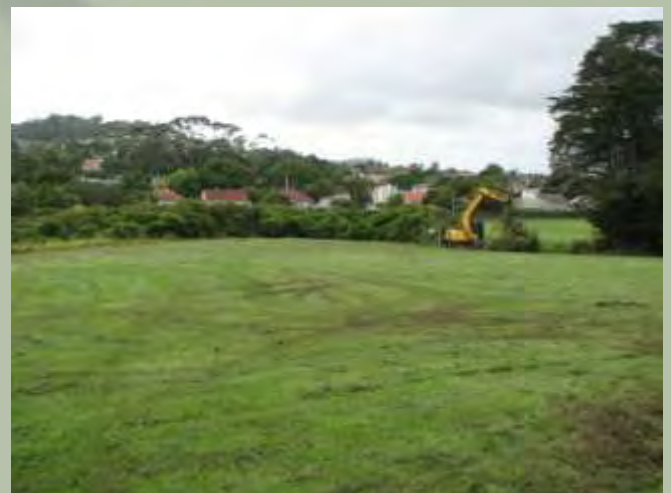
The clearing starts.
