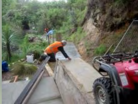
Before, during and after ... Repairs were made in October to the Plane Tree Bridge boardwalk, which had been slowly sinking down towards the creek - thanks to Auckland Council for this great improvement.
