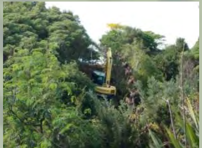
Site prep for replanting in drilling sites. Watch out below!
